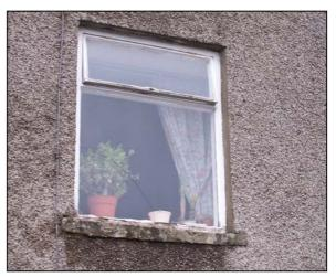
Figure 92. Decaying window and lintel
