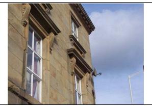
FIGURE 92. MOULDED CORNICES ON SCROLLED BRACKETS CHARACTERISE THE FIRST FLOOR LEVEL
