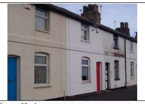
FIGURE 89. A CONTINUOUS SILL BAND RUNS THE LENGTH OF THE TERRACED ROW AT FIRST FLOOR LEVEL
