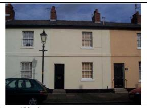
FIGURE 133. A CONTINUOUS SILL BAND RUNS THE LENGTH OF THIS TERRACE AT FIRST FLOOR LEVEL
