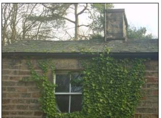
Figure 59. Example of slate roofing
