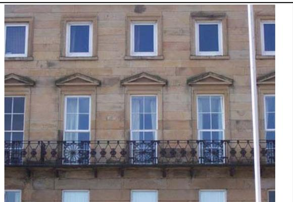
FIGURE 50. BALCONIES WITH ELABORATE CAST IRON BALUSTRADES CHARACTERISE THE FIRST FLOOR
