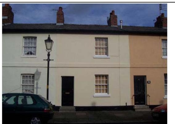
FIGURE 133. A CONTINUOUS SILL BAND RUNS THE LENGTH OF THIS TERRACE AT FIRST FLOOR LEVEL
