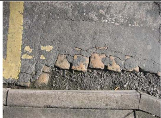
FIGURE 57. STONE SETTS ARE EVIDENT BETWEEN THE TARMAC ON AUGHTON STREET
