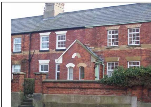
FIGURE 33. MANY TRADITIONAL SASH WINDOWS HAVE BEEN REPLACED BY MODERN UPVC FRAMES
