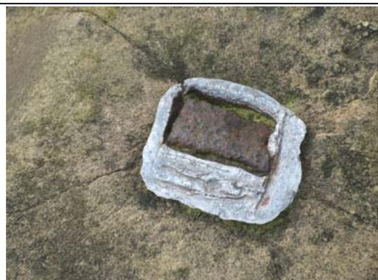
FIGURE 26. CAST IRON RAILINGS ONCE SURMOUNTED THE STONE WALL TO THE NORTH OF THE MOUNT
