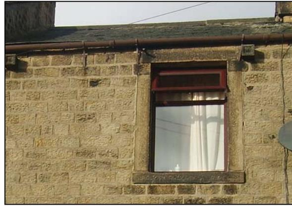
Figure 64. Modern timber replacement window
