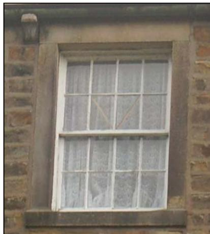
Figure 61. Original 'eight over eight' arrangement sash window
