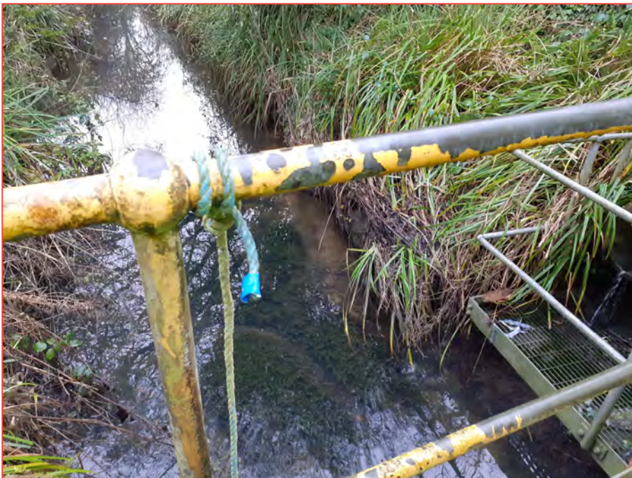
Photo 18: RB06 Round 4 – Royles Brook, Penstock, final location of Royles Brook prior to leaving Hillhouse complex
