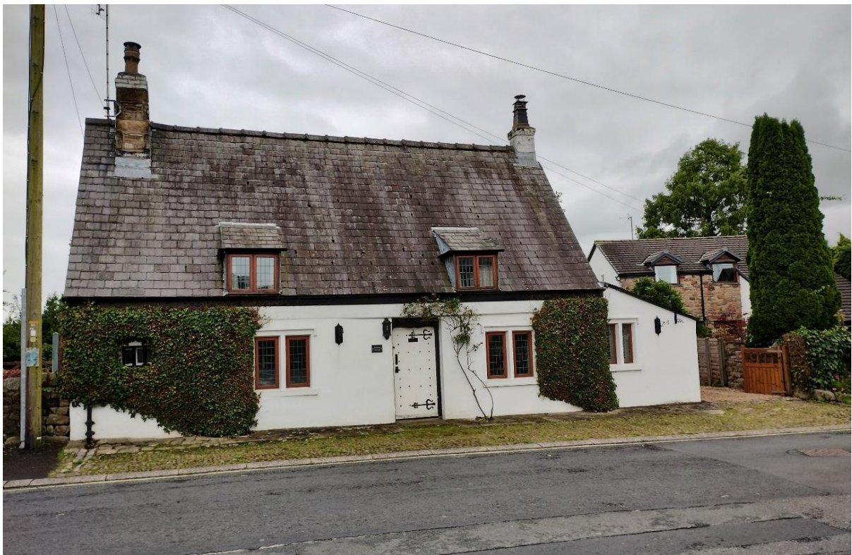
Figure 25: The Grade II listed C17 Primrose Cottage with fire window (left)
