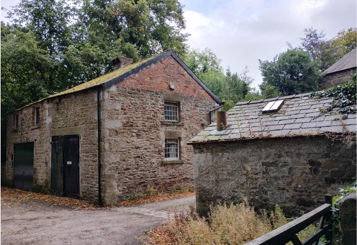
Figure 22: Outbuildings to Springfield House
