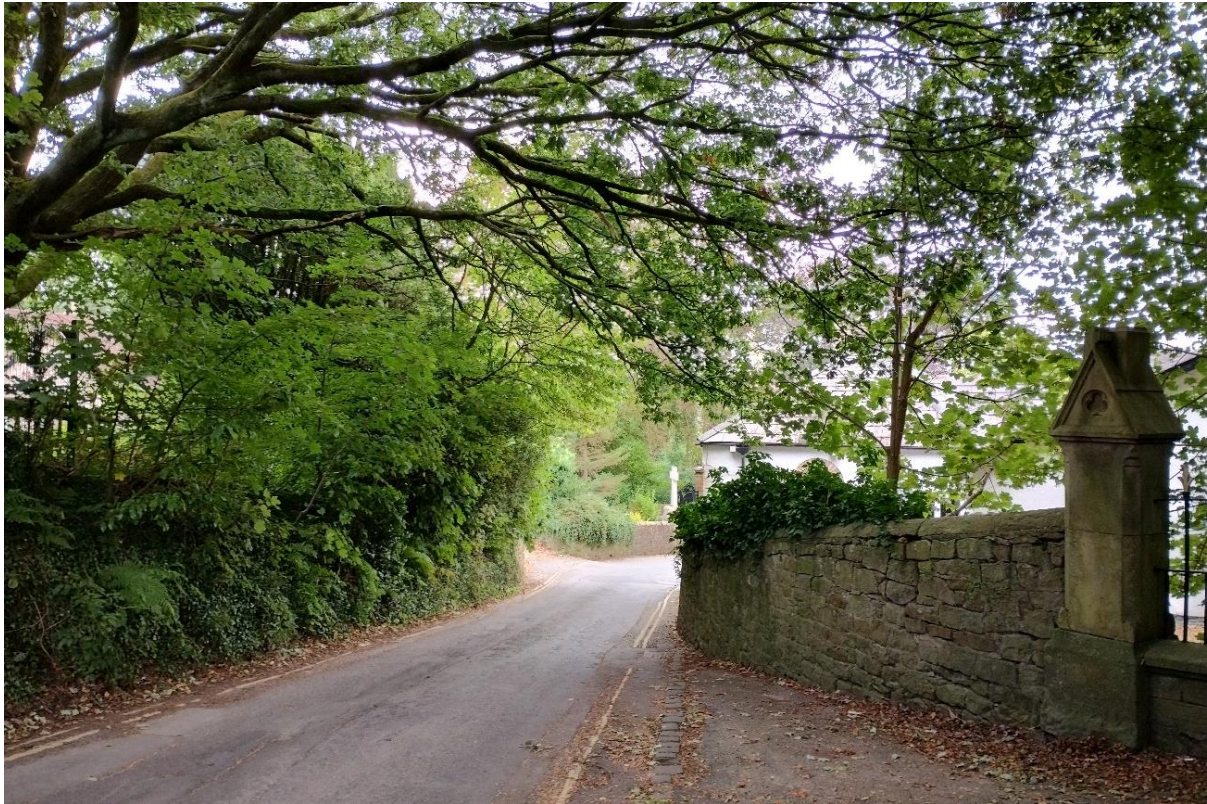
Figure 13: Sandstone walling enclosing Snowhill Lane
