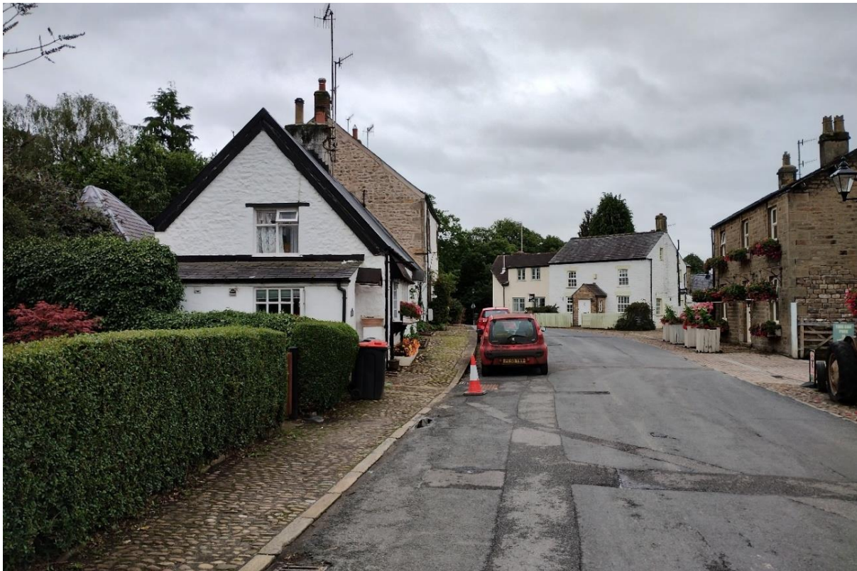
Figure 28: Formerly thatched cottages (left) with steep pitches; where chimney have been removed erodes character.
