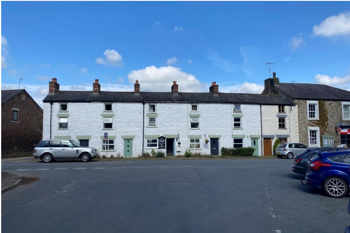
Figure 3: Uniform 18th century workers' cottages
