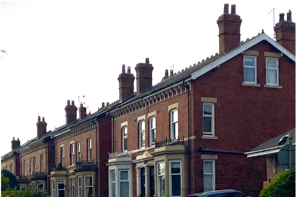
Figure 37: Roofscape along Victoria Road
