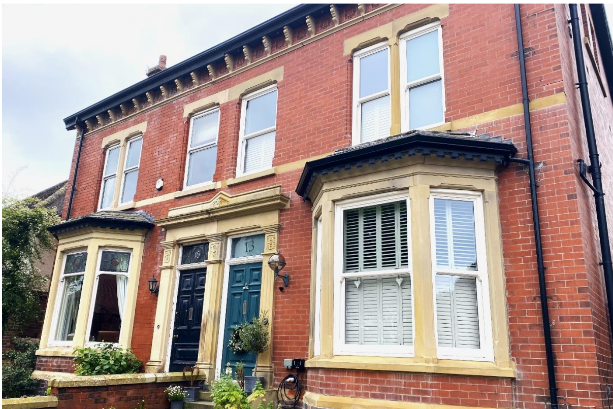
Figure 4: Brick built semi-detached villas on Victoria Road
