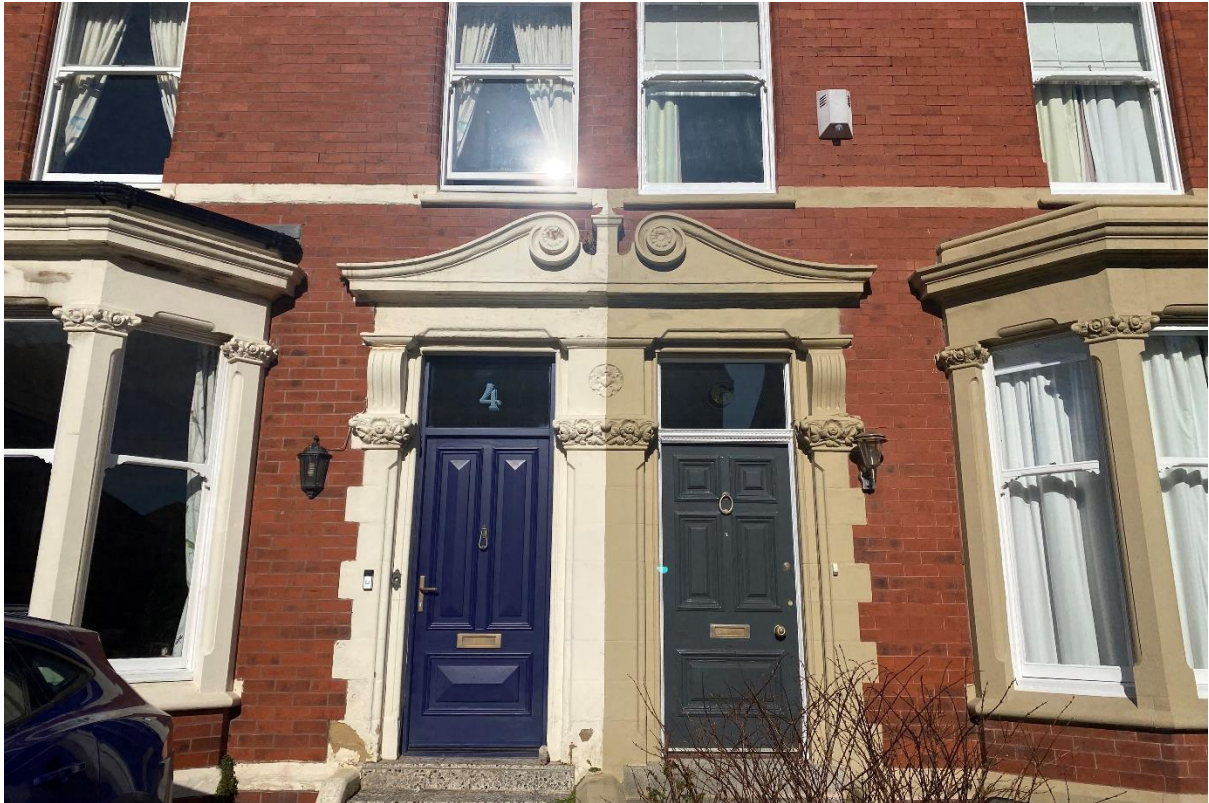
Figure 30: Masonry detail of 4 and 6 Victoria Road
