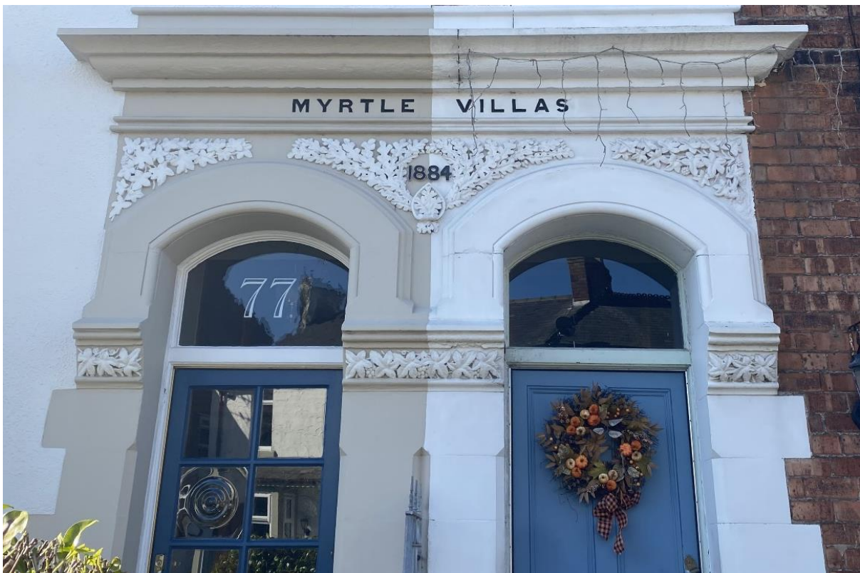
Figure 31: Masonry detail of 75 and 77 Station Road
