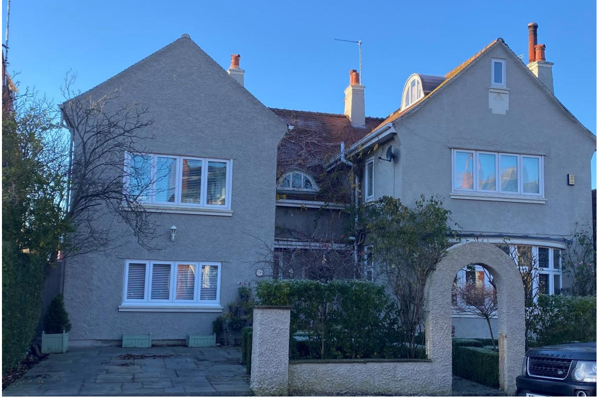
Figure 36: Eyebrow dormers on 14 Lockwood Avenue
