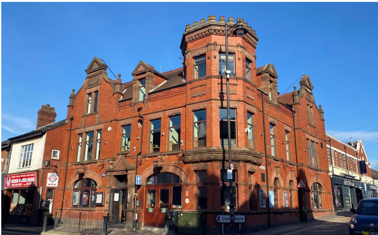
Figure 8: The former Ship Inn
