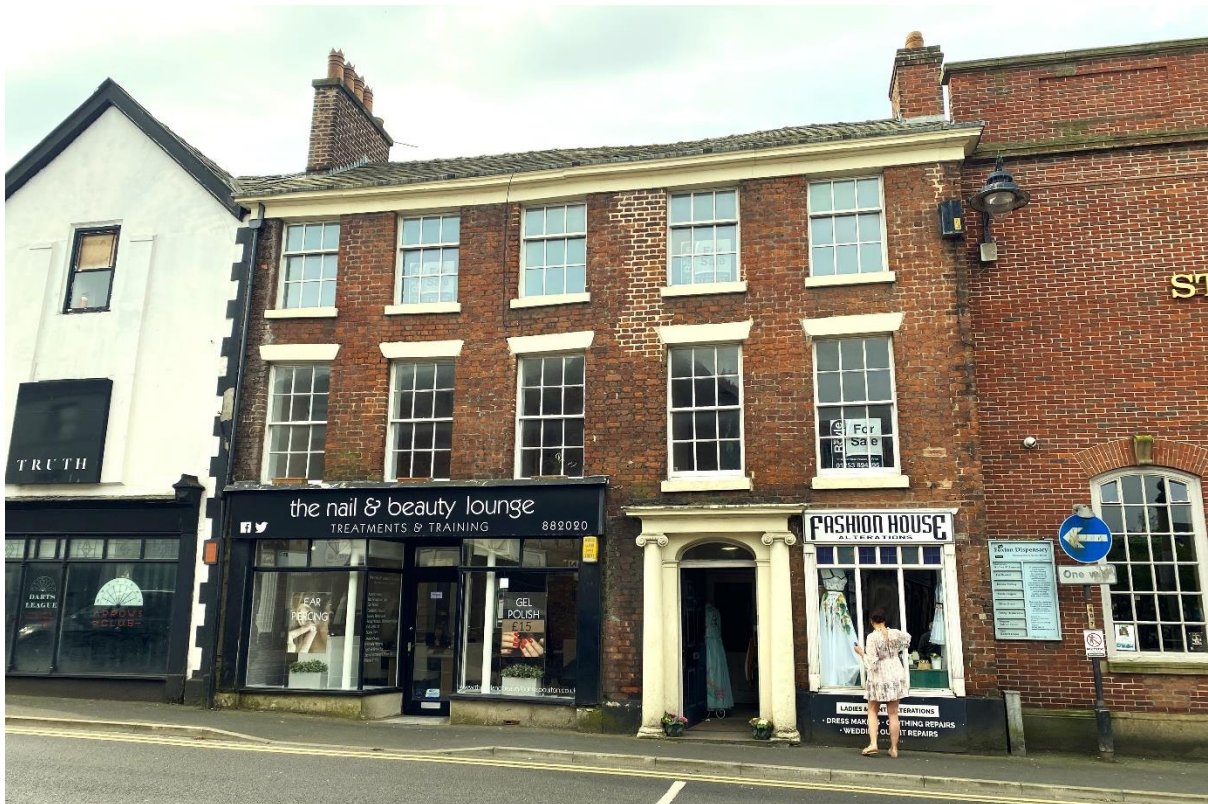
Figure 16: Grade II listed 25 - 31 Market Place
