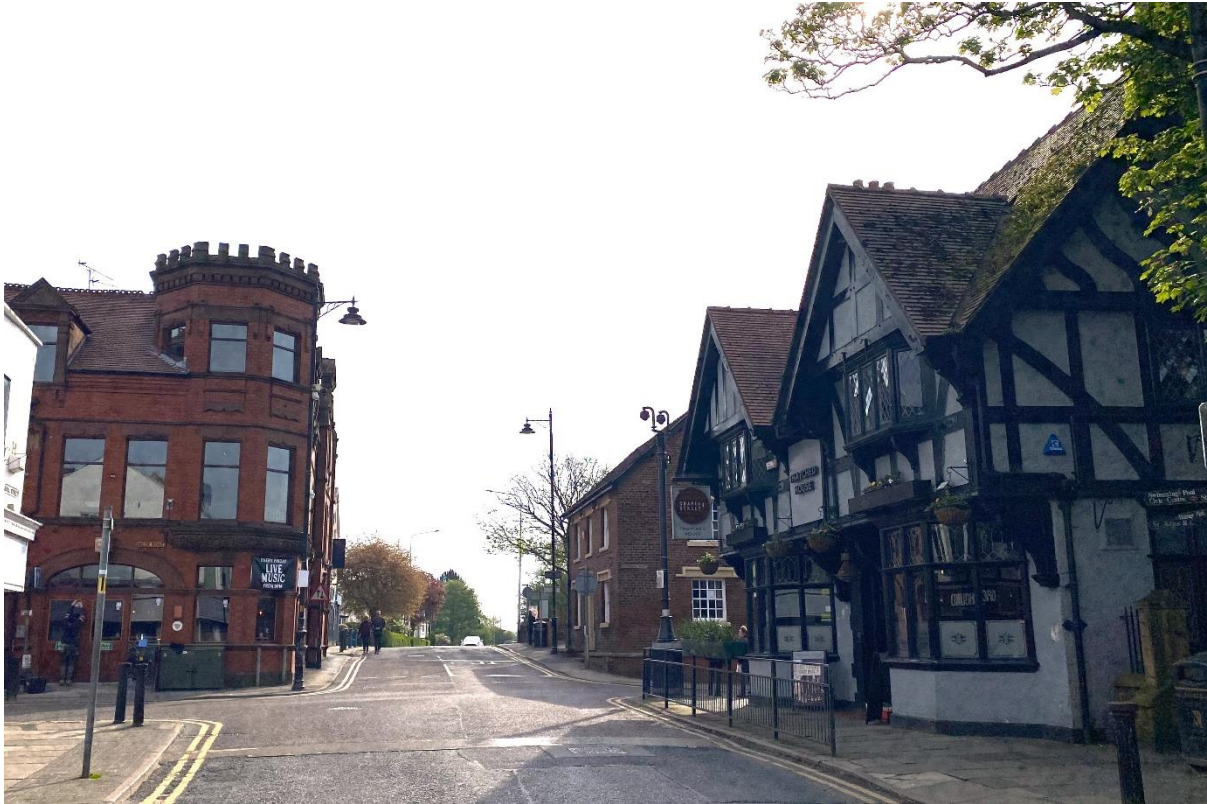
Figure 3: The former Ship Inn, the Thatched public house and the Grade II listed 1 Vicarage Lane
