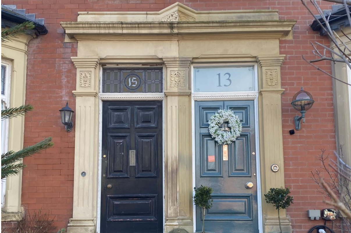
Figure 28: Timber panelled doors on Victoria Road
