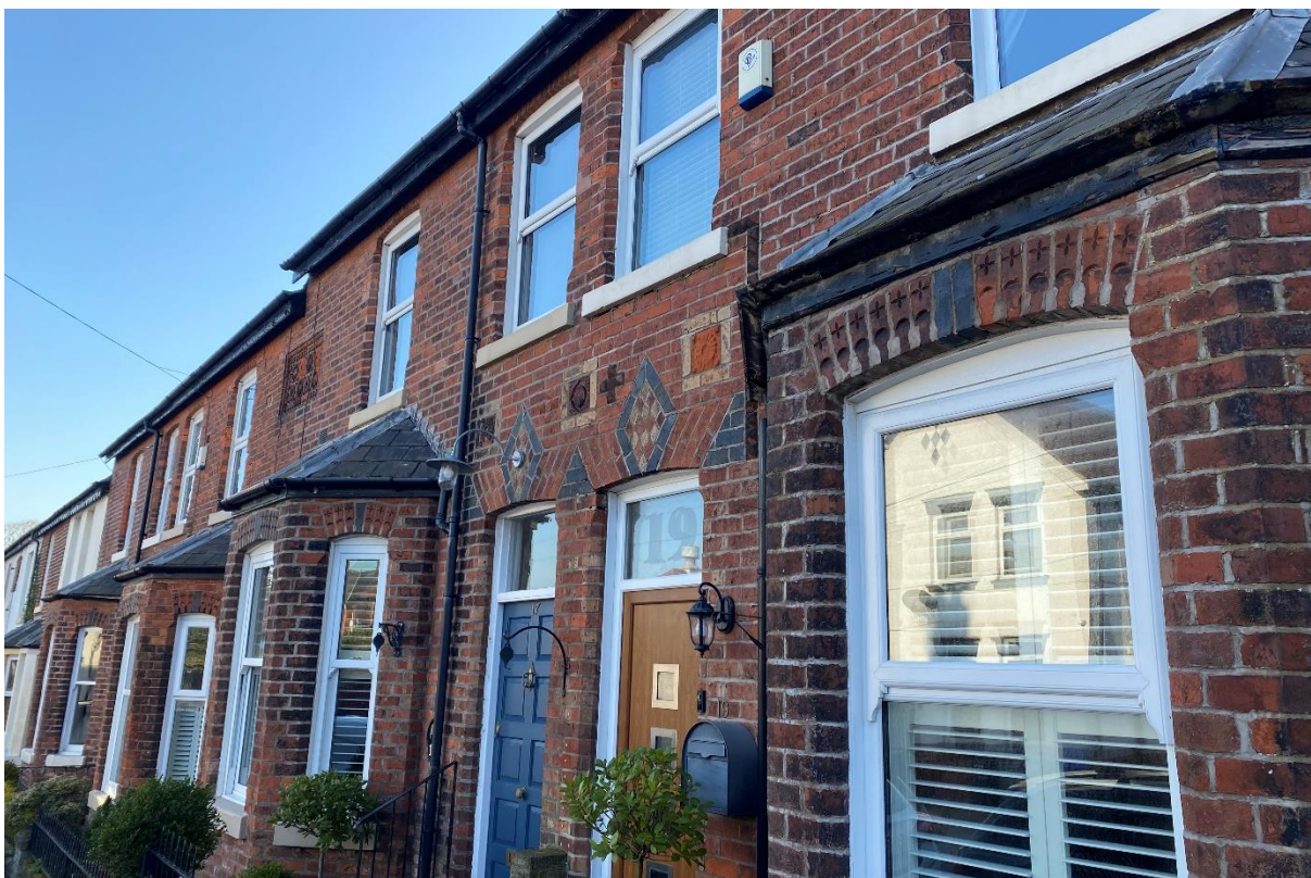
Figure 33: Detail of brickwork on terraced housing along Elletson Street
