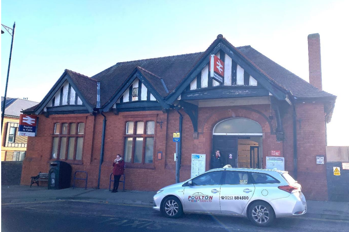
Figure 24: Poulton-le-Fylde railway station
