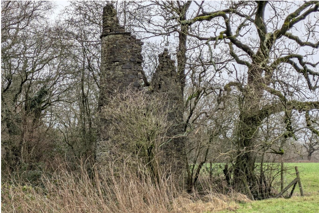
Figure 20: The remains of the chimney to the gas plant, which forms part of the Scheduled Monument.
