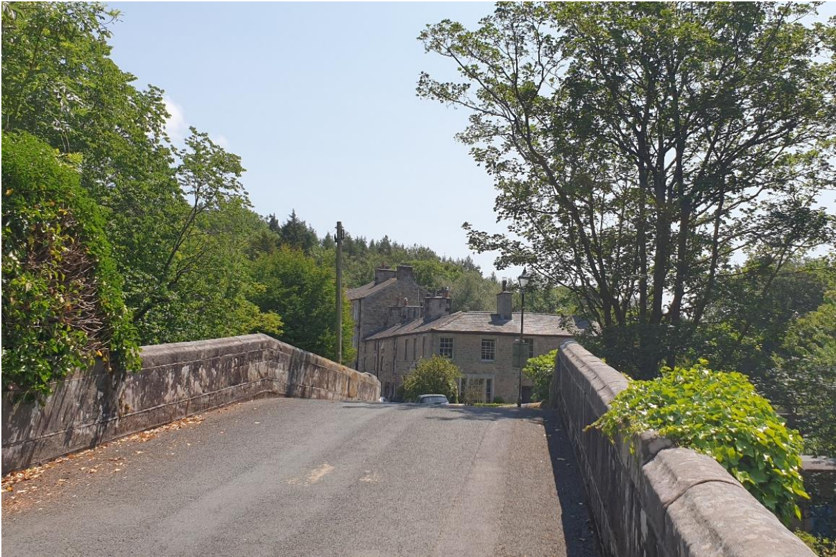
Figure 1: Dolphinholme Bridge and views south into the village
