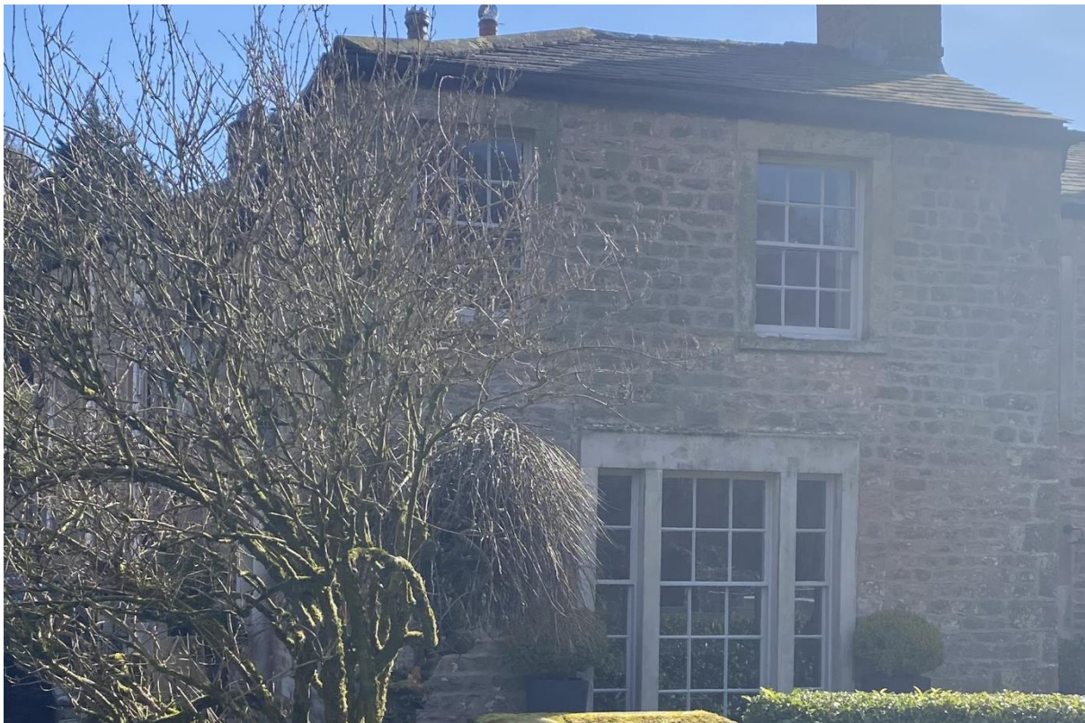
Figure 22: Tripartite sash window to the side of Derham house
