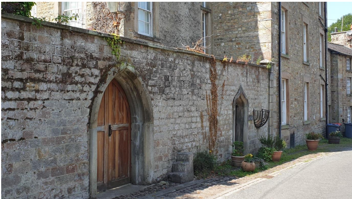
Figure 13: The door openings in the Grade II listed wall adjacent to Old Mill House.
