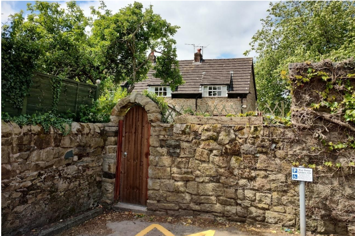
Figure 18: Weind walls to the rear of Barnacre view adapted to form property boundaries
