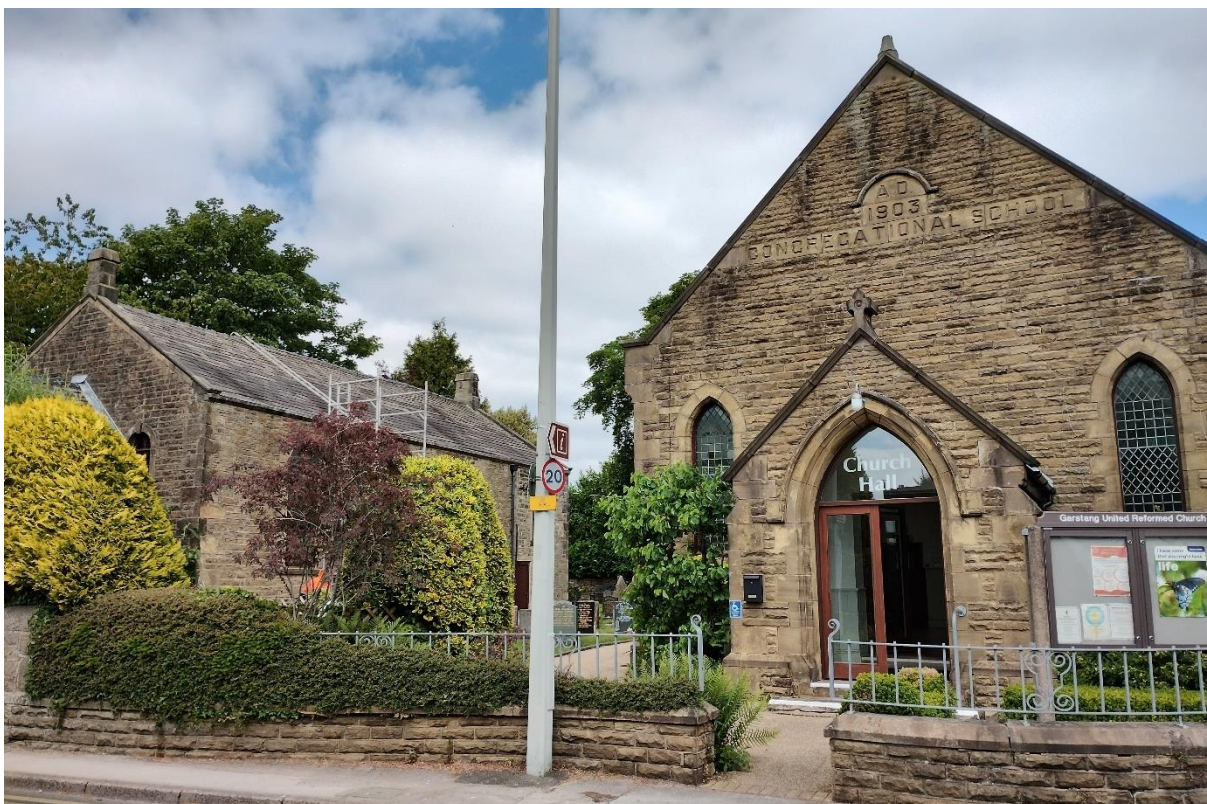
Figure 19: Curved walls to the United Reformed Church and Congregational Chapel
