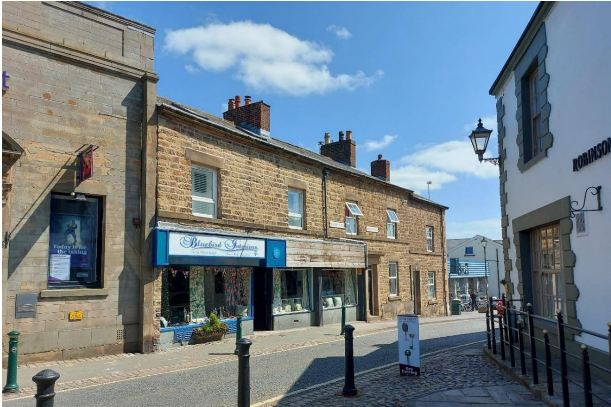
Figure 1: Pinch points along High Street
