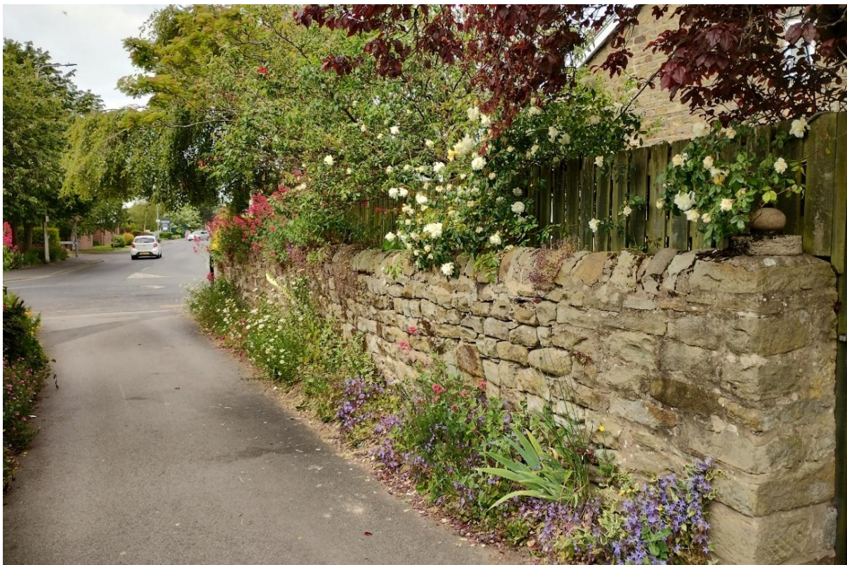
Figure 17: Historic walling adapted to create property boundaries
