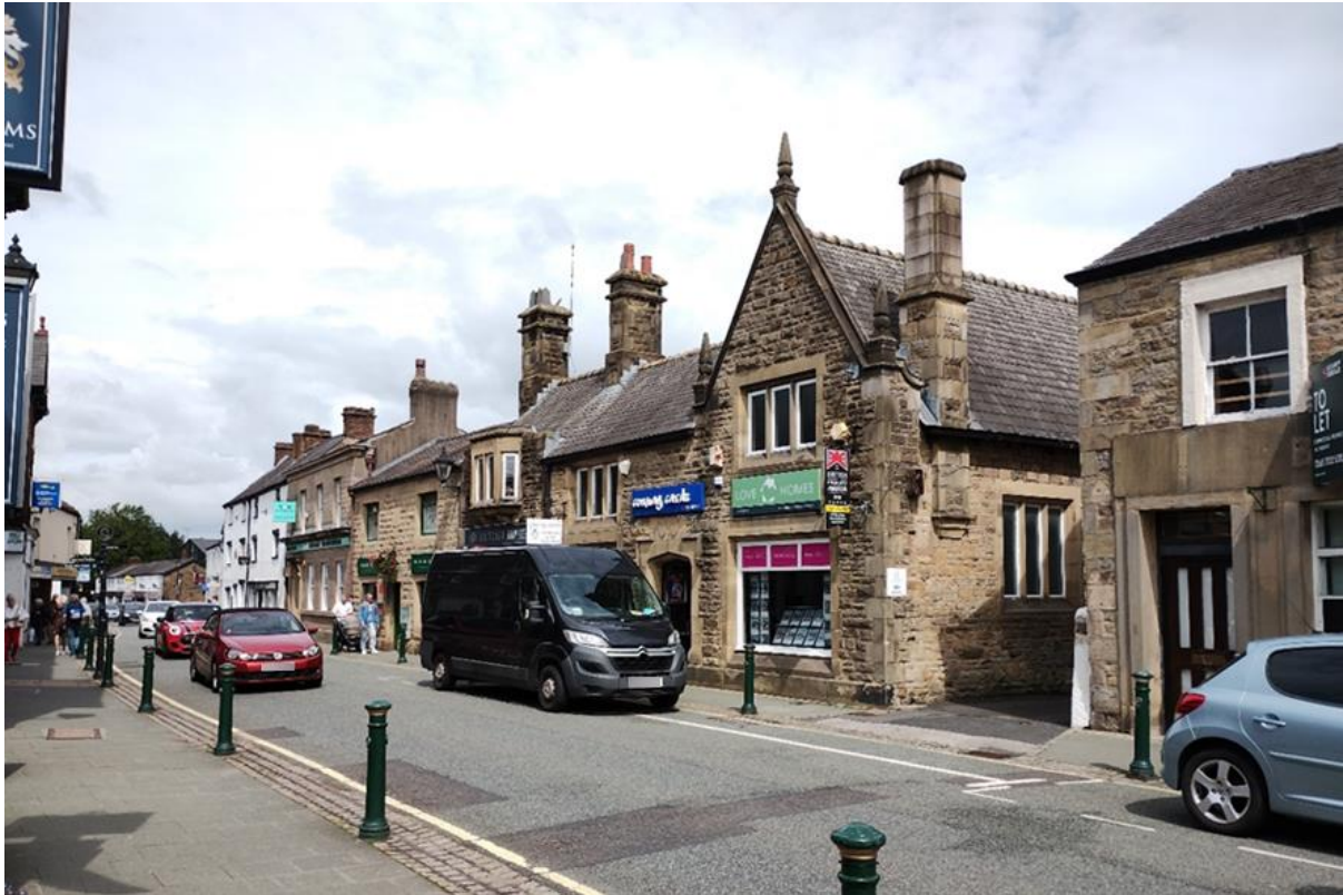
Figure 10: Views along High Street encompassing varied rooflines
