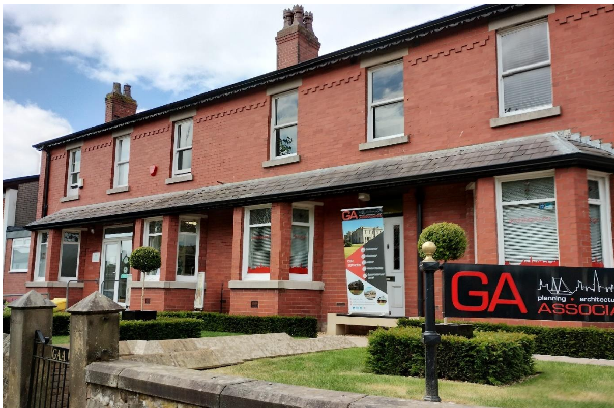
Figure 29: Dentilated brickwork at Croston Villas
