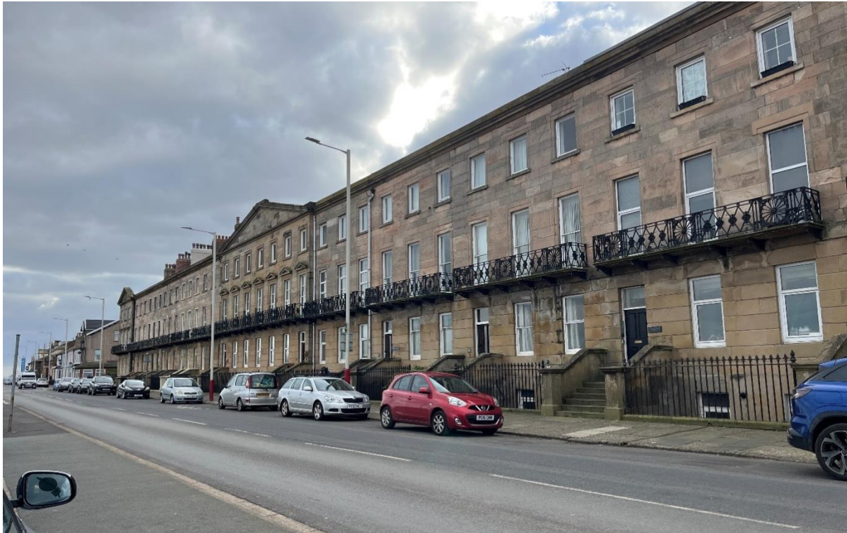
Figure 9: View along the formal frontage to Queen's Terrace
