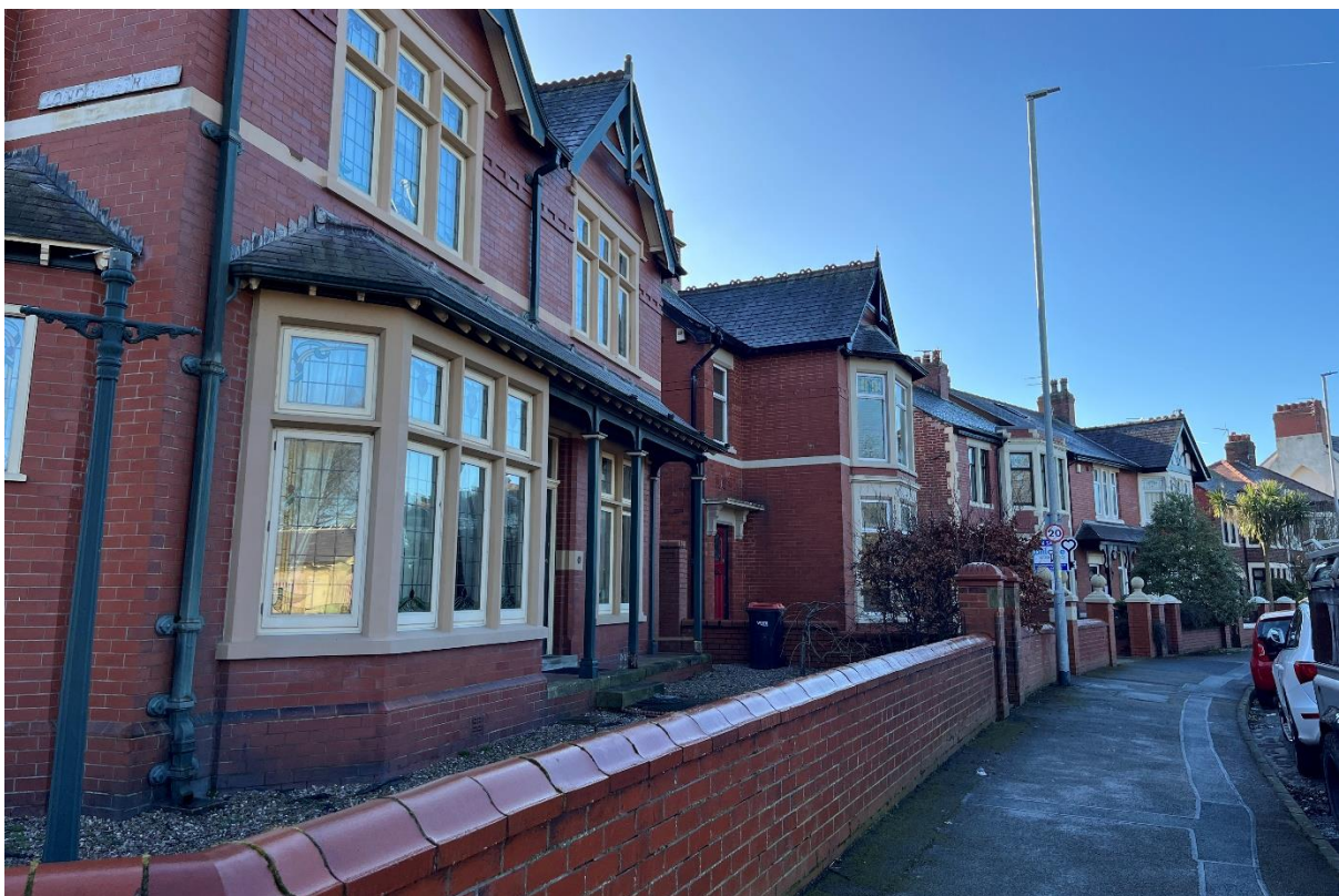
Figure 18: Mix of red brick front garden walls and gate piers to residential properties
