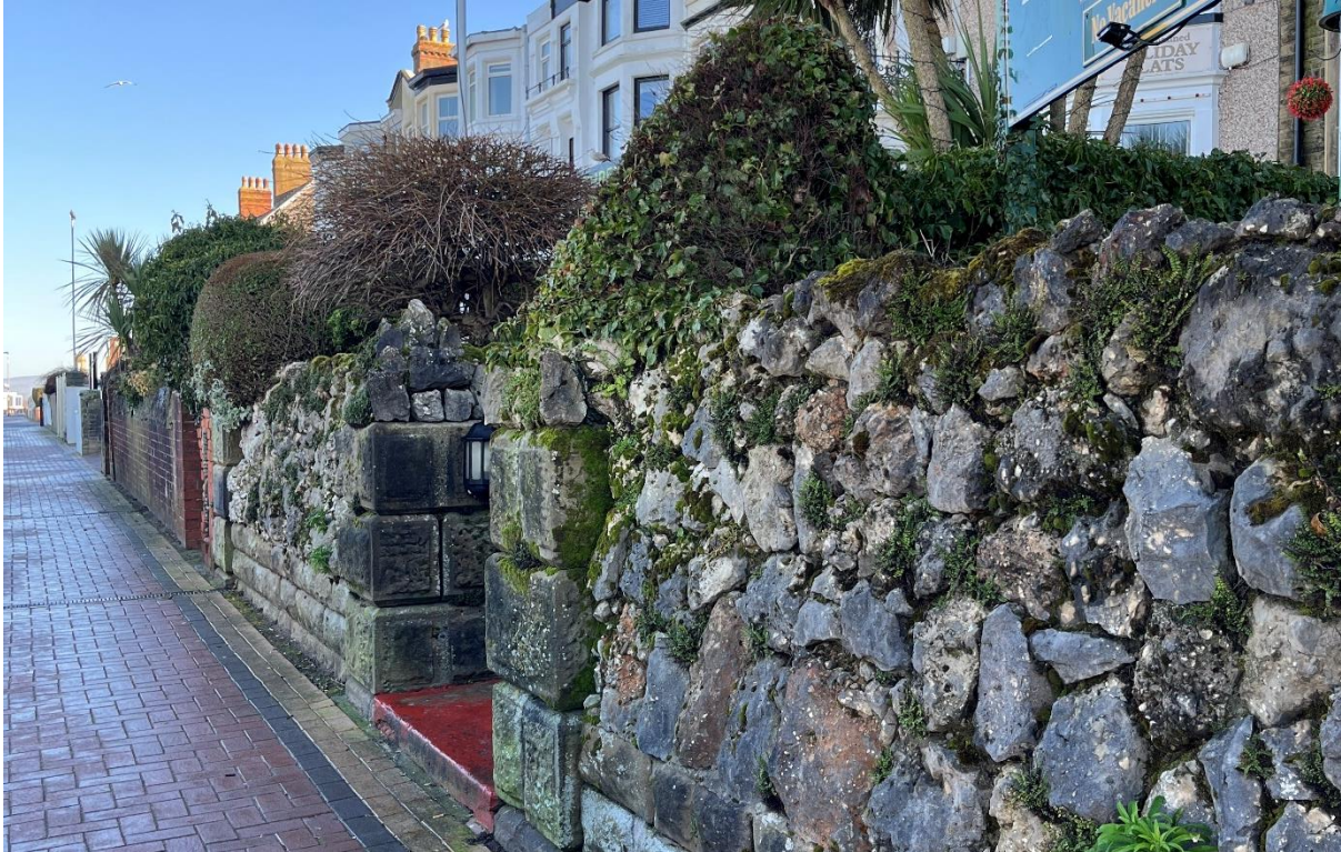
Figure 17: Rubble stone walls outside 29 The Esplanade
