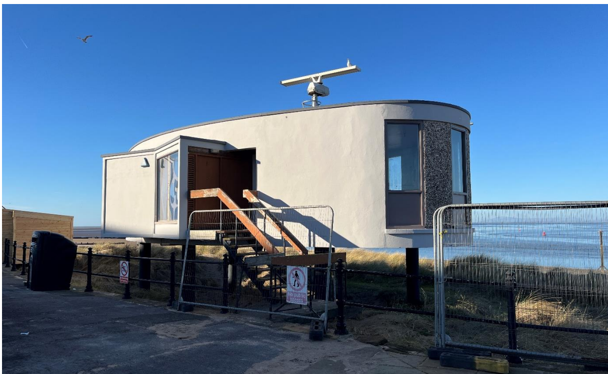
Figure 7: The Grade II listed Fleetwood Radar Training Station
