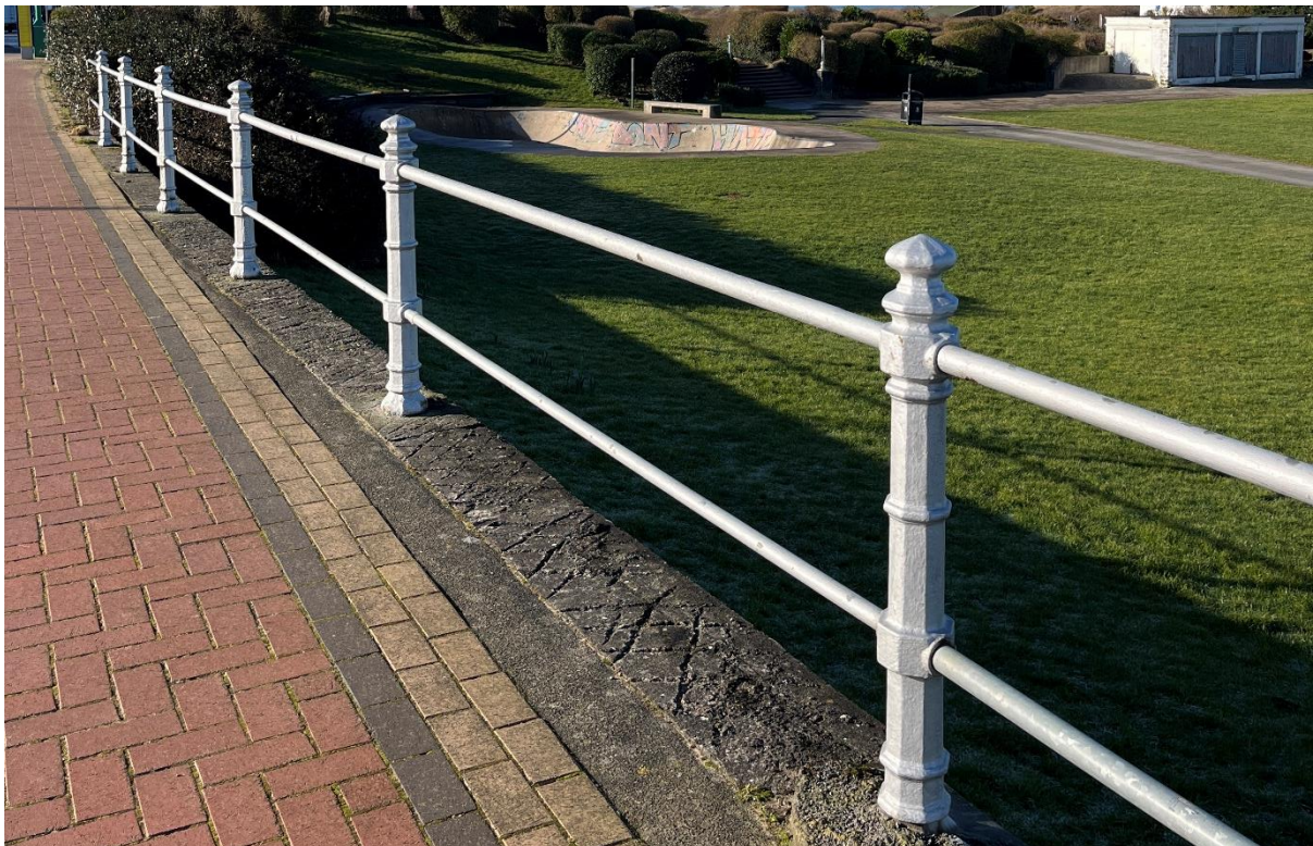
Figure 16: Cast iron post and rail fencing provides an open edge to the Marine Hall Gardens
