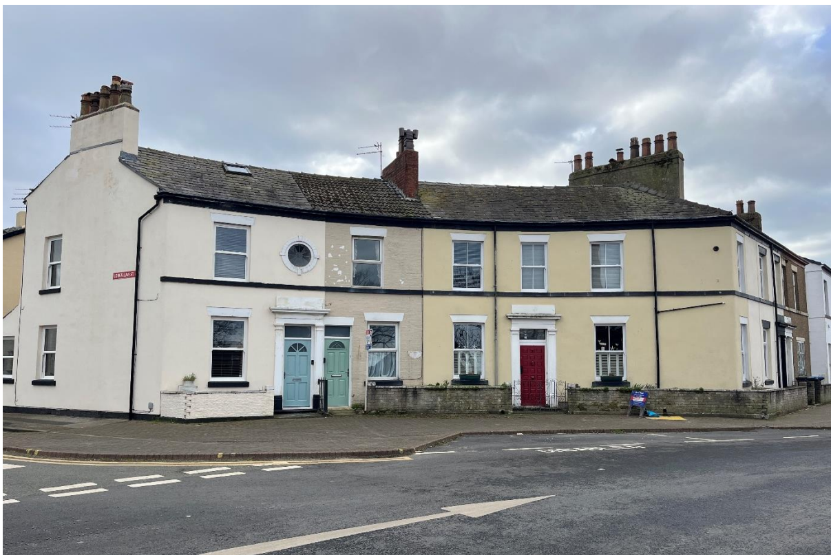
Figure 36: The Grade II listed 1-9 Pharos Terrace
