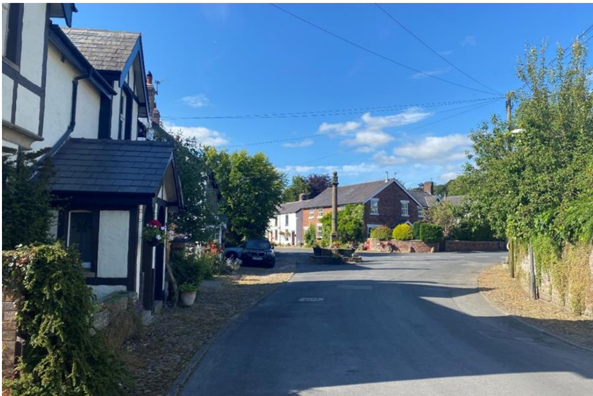
Figure 6: The Village Cross and cobbled paving provide a focal point at the central junction of the village
