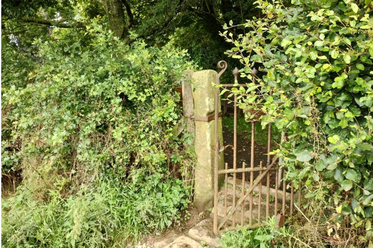
Figure 13: Cast and wrought iron gate to the footpath to the south of the churchyard
