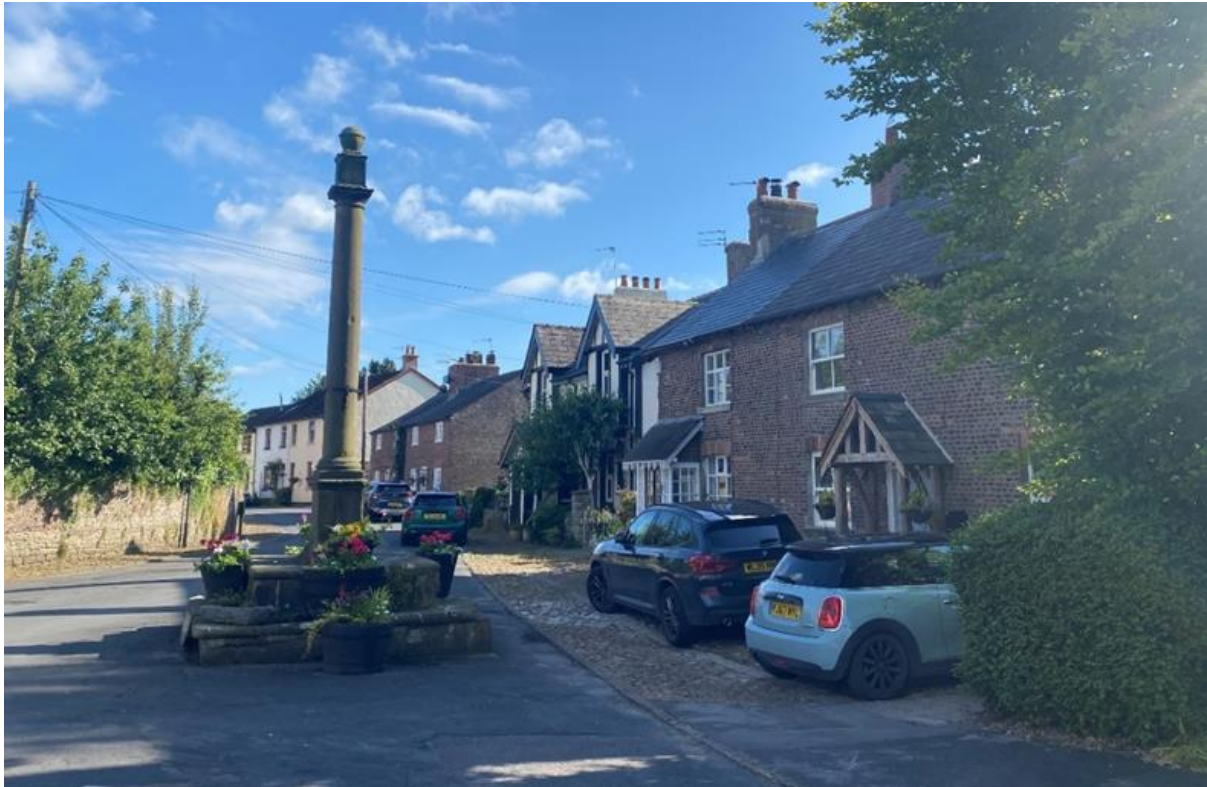
Figure 7: Views south towards the varied roofscapes of The Green
