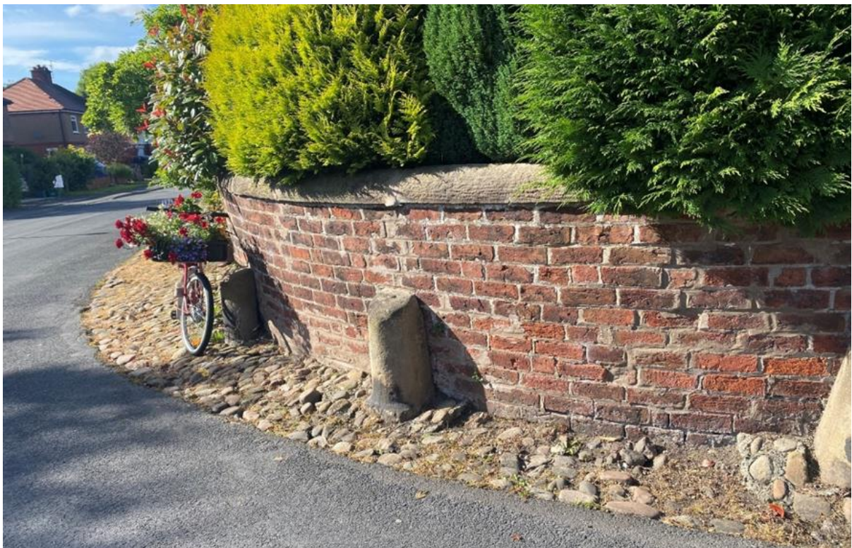
Figure 14 Handmade brick boundary wall and guardstones complemented by cobbled paving at the junction of Ainspool and The Green
