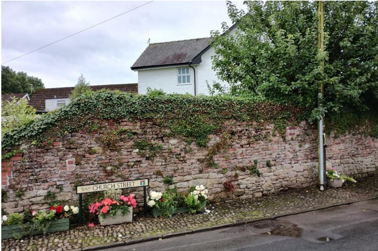
Figure 15 The stone and brick wall along Church Street complemented by cobbled paving
