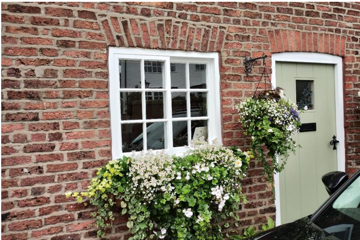
Figure 23 A Yorkshire sliding sash
