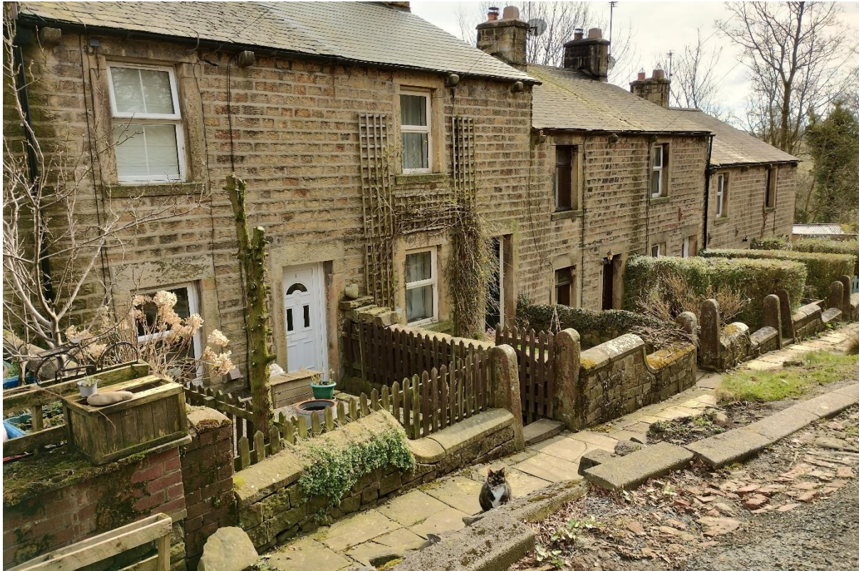
Figure 15: Stone boundary walls and sandstone flags along Albert Terrace
