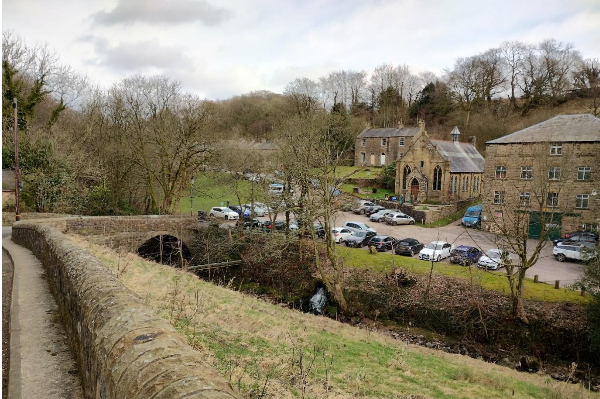
Figure 3: The Bridge, Methodist Chapel, Mill, and Mount Pleasant
