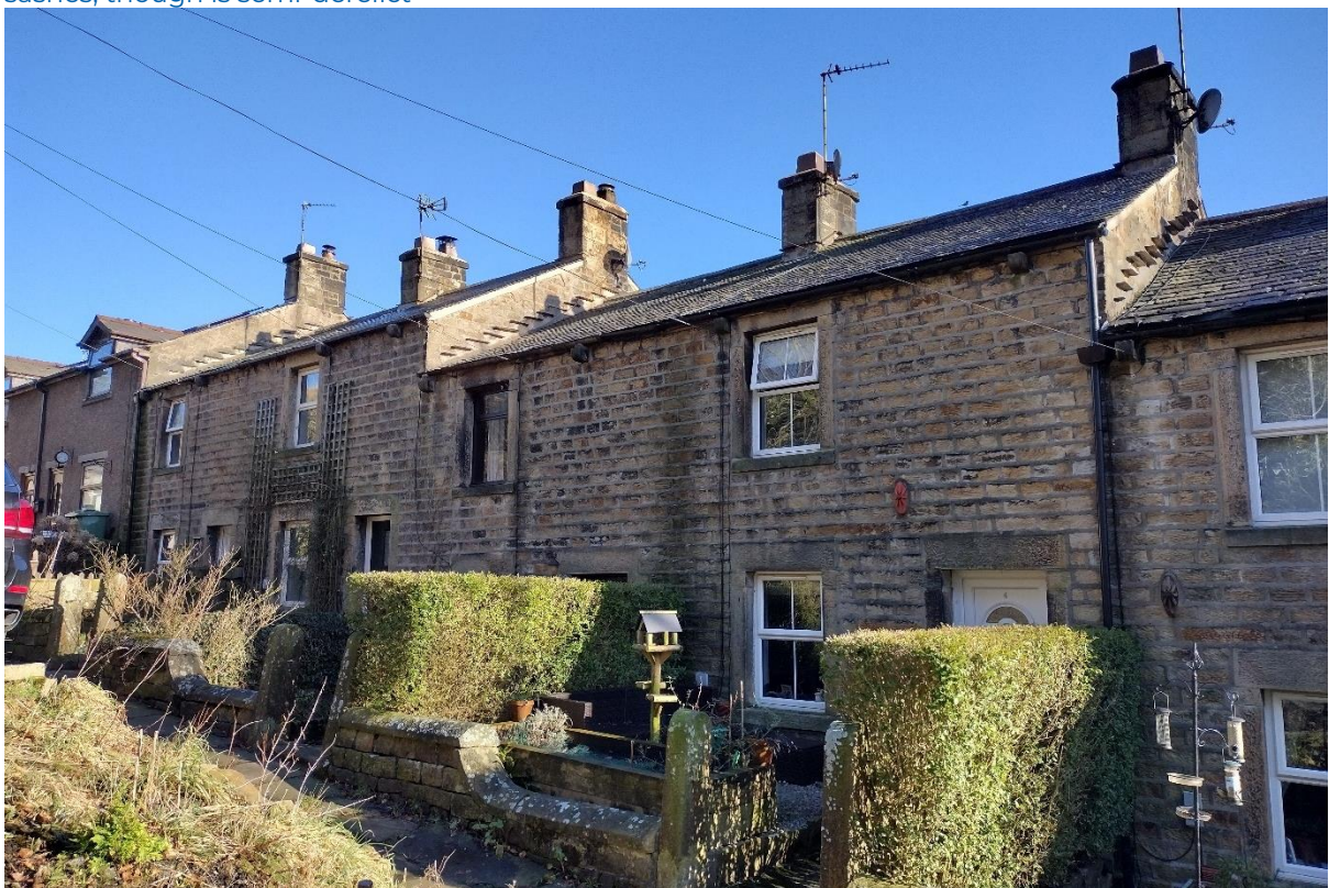
Figure 23: Regularly spaced chimneys and drip stones to gable ends
