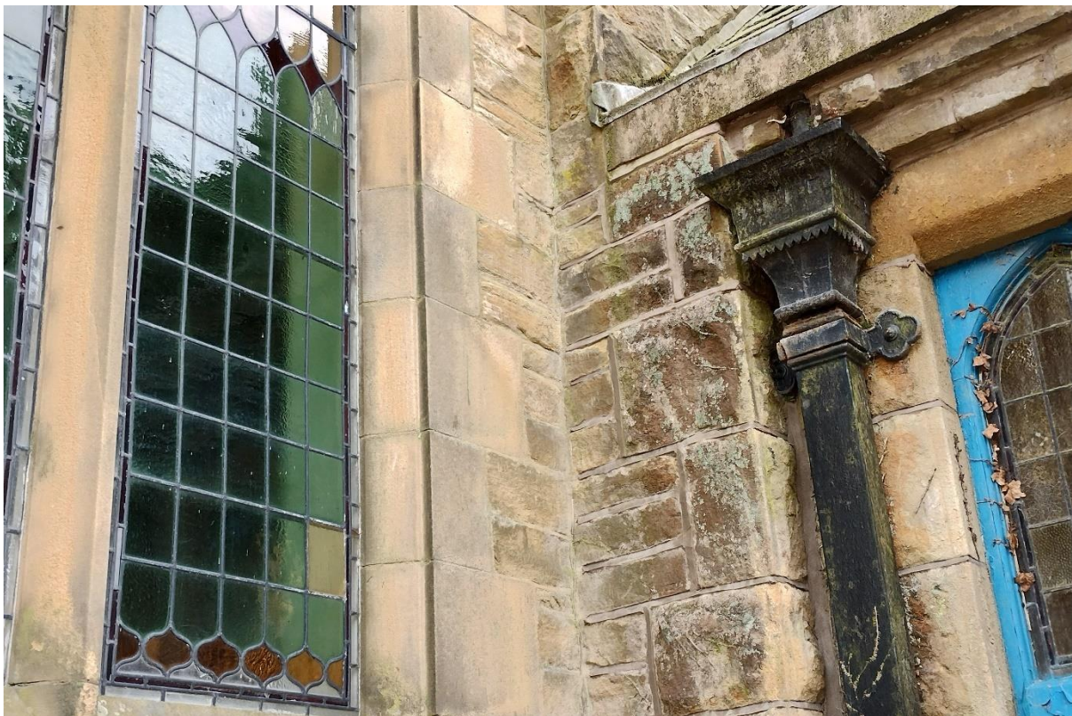
Figure 19: Leaded lights and an original cast iron downpipe at the Wesleyan Methodist Chapel
